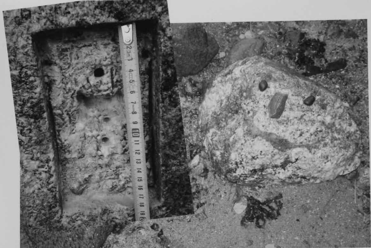
The slot for EWS1 was fitted by hand. Work on slot finished 3.8.2012. Some random faces where spotted on site.
